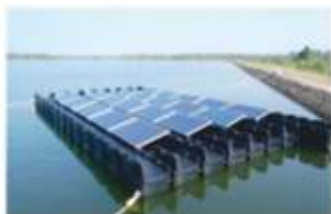
5kWp pilot plant of floating Solar PV System installed @ Rajiv Gandhi Combined Cycle Power Plant (RGCCPP), Kayankulam, Kerala
