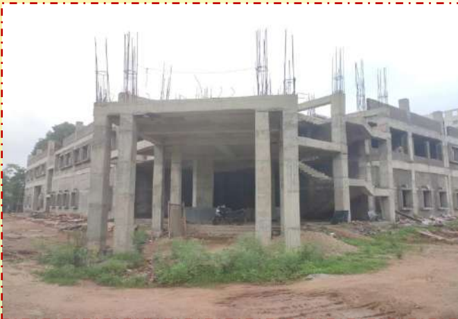
Construction work of vertical extension (Additional 2 floors) on existing Boys Hostel is under final stage of completion at Aurangabad centre.
